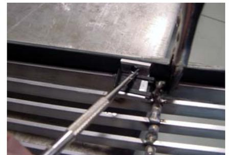
**STEP 9** Insert and center the billet grille as shown with the short edges of the brackets even with the back edges of the shell, then clamp in place and mark the slotted hole locations and drill a 1/8" hole 1/8" from the edges of the plastic on the center line of the slotted hole.
